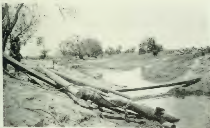
BRIDGE BUILDING. MAHOGANY BALKS; TELEGRAPH WIRE; DOGS OF LOCAL IRON; AND STRIPS OF SPLIT PALM.
